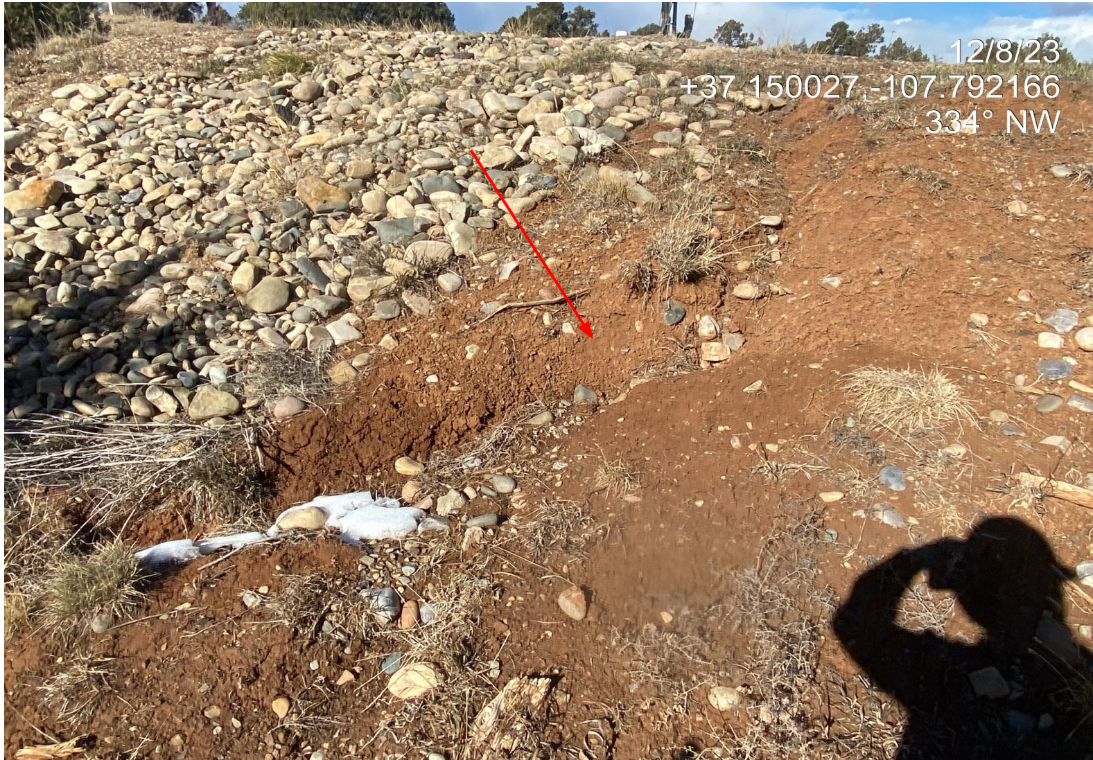
Photo 2. View of rill/gully erosion forming in the western portion of the interim reclamation area. Additional erosion BMPs are needed for this area.
