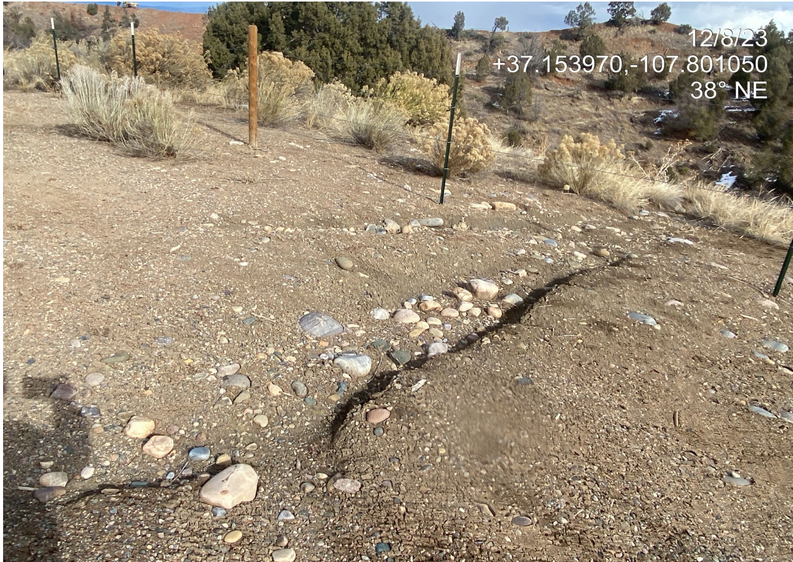
Photo 2. View of rill erosion forming on the eastern edge of the disturbance. Additional erosion BMPs needed in this area.
