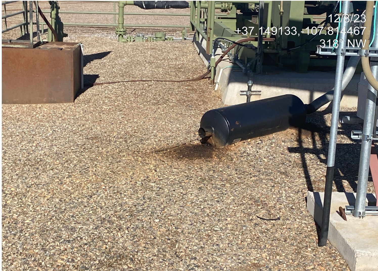
Photo 3. View of stained soils near muffler on location.
