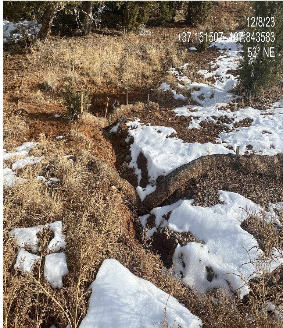
Photo 2. View of failing stormwater erosion BMPs observed in the northern interim reclamation area adjacent to the access point/entrance. Additional stabilization is needed in this area.
