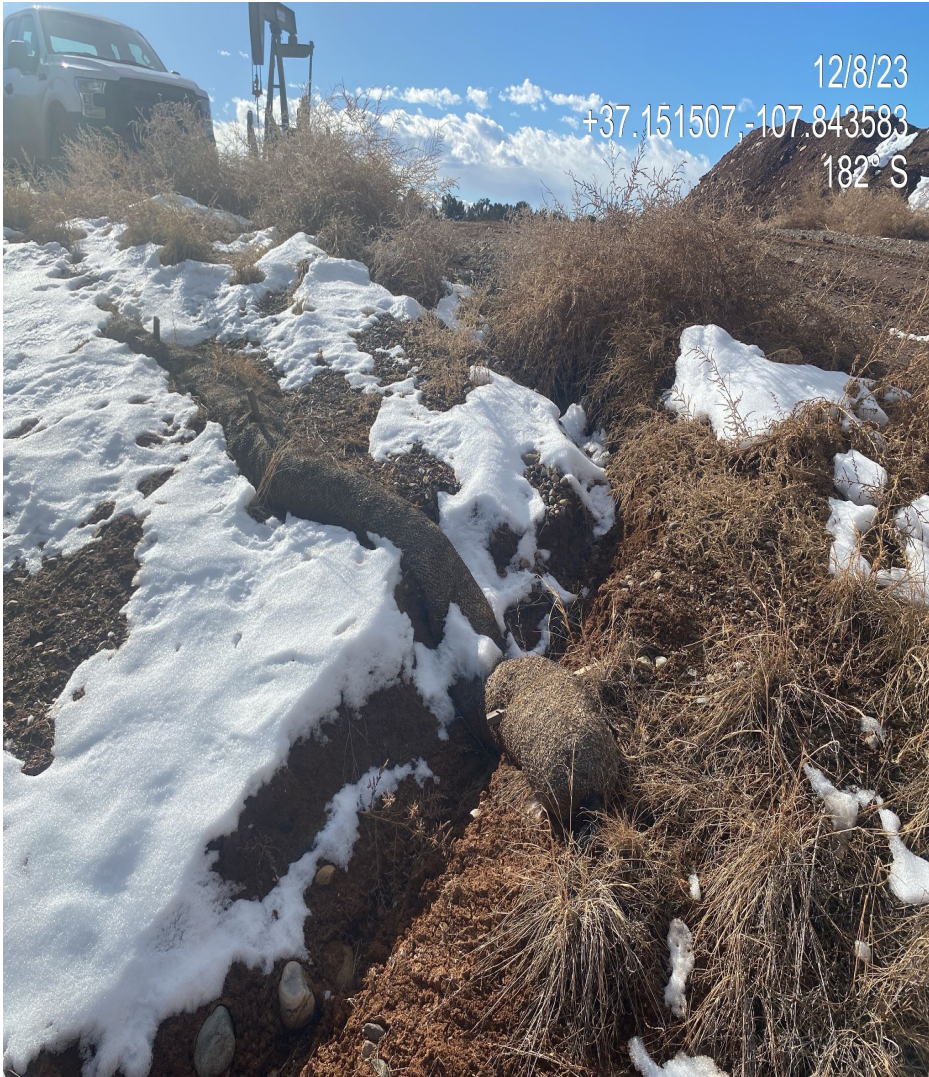
Photo 2. View of failing stormwater erosion BMPs observed in the northern interim reclamation area adjacent to the access point/entrance. Additional stabilization is needed in this area.
