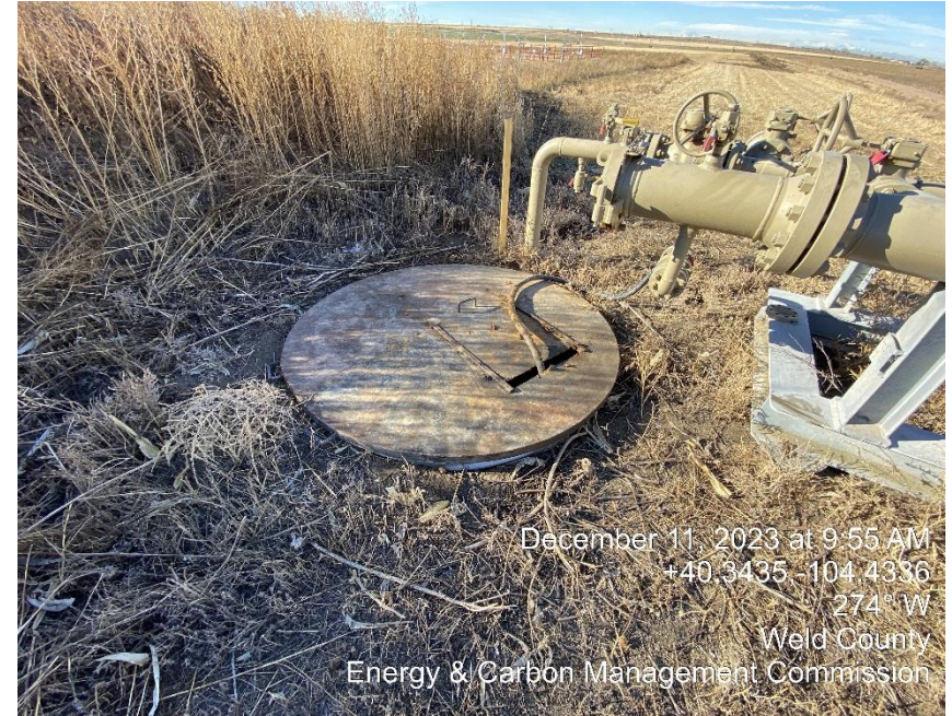
Pit needs berms/ capacity sign/ NFPA placard and pigging waste removed.
