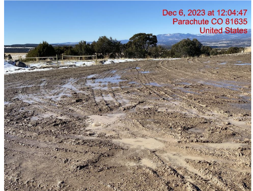
Insufficient Vehicle Tracking BMPs at Location Entrance/Exit – Photo #08033
