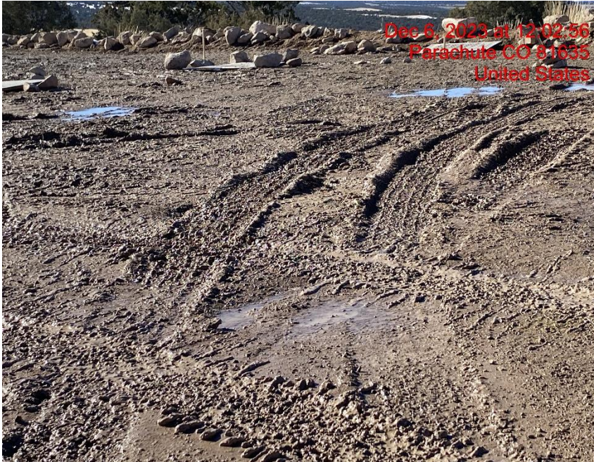
Lack of Stabilization – Photo #08028
