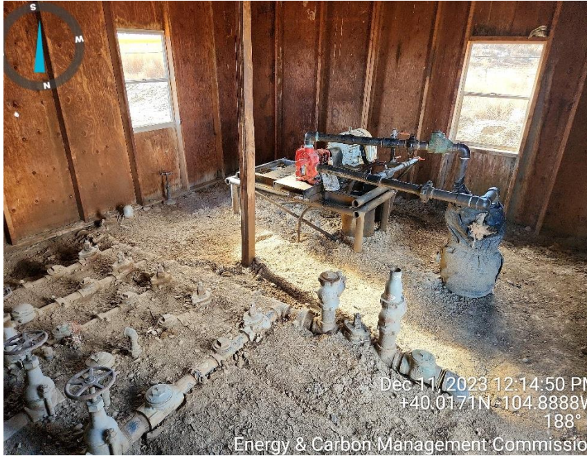
Photo 7 valve manifold and circulating pump equipment
