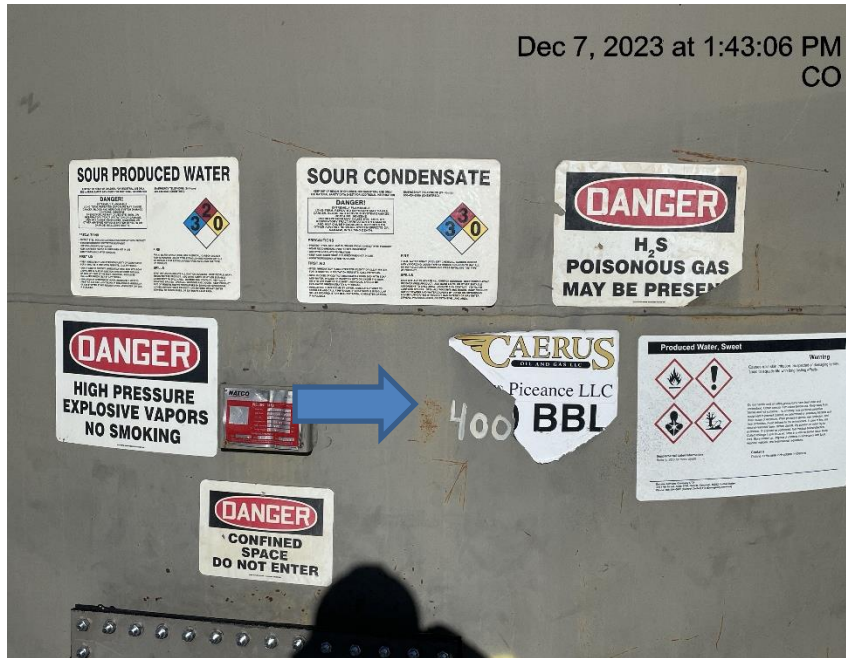
Photo # 8917 Tank labeled damaged & missing required information
