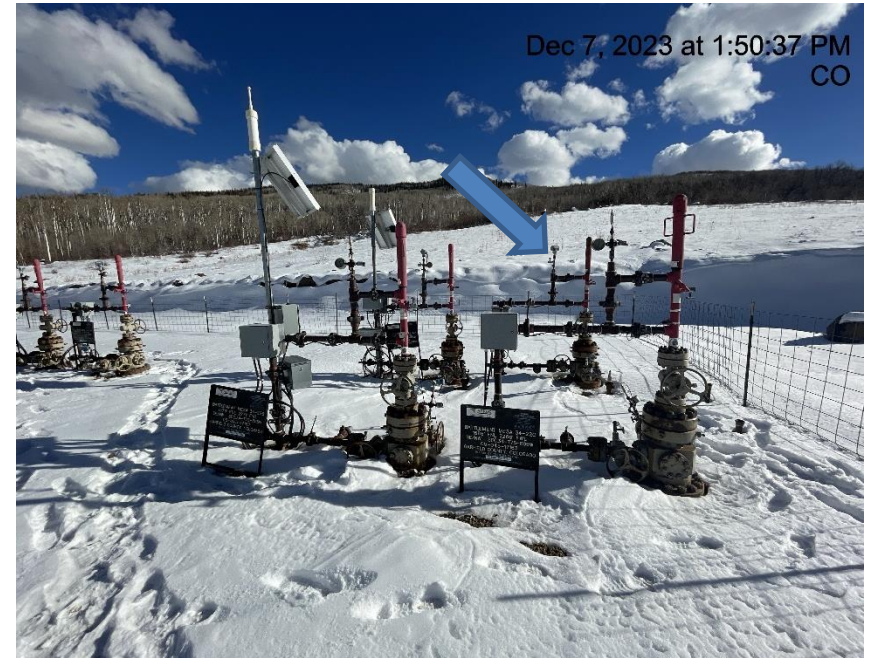
Photo # 8924 Wellhead lacks signage
