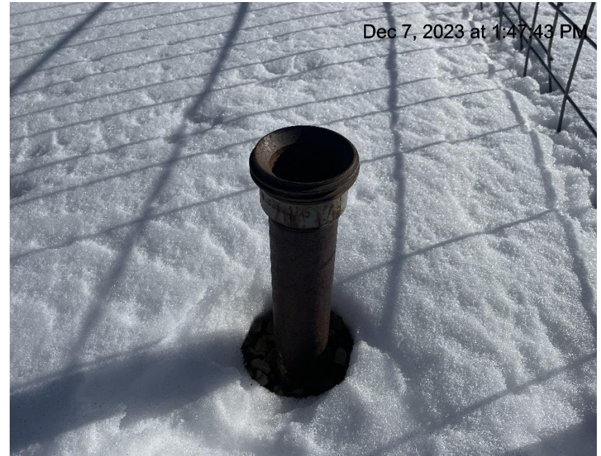
Photo # 8920 Open ended piping/wildlife hazard
