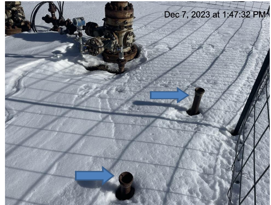
Photo # 8918 Open ended piping/wildlife hazards
