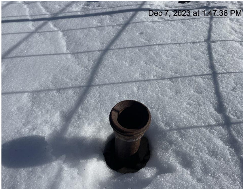
Photo # 8919 Open ended piping/wildlife hazard
