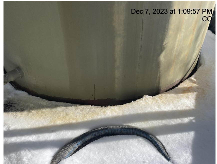
Photo # 8845 Staining in secondary containment
