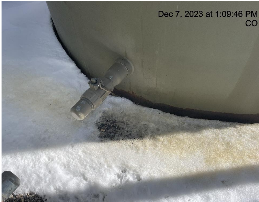
Photo # 8844 Staining in secondary containment
