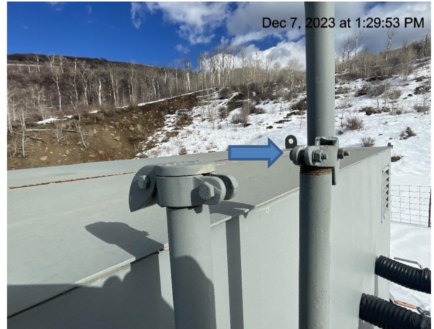
Photo # 8886 PRV vent line lacks cap
