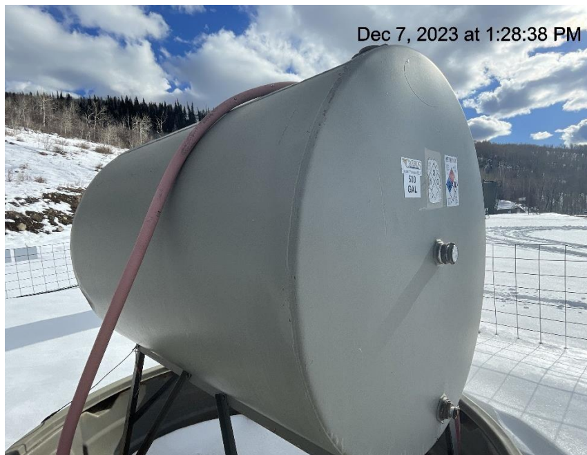
Photo # 8883 Methanol tank improperly labeled/lacks required information
