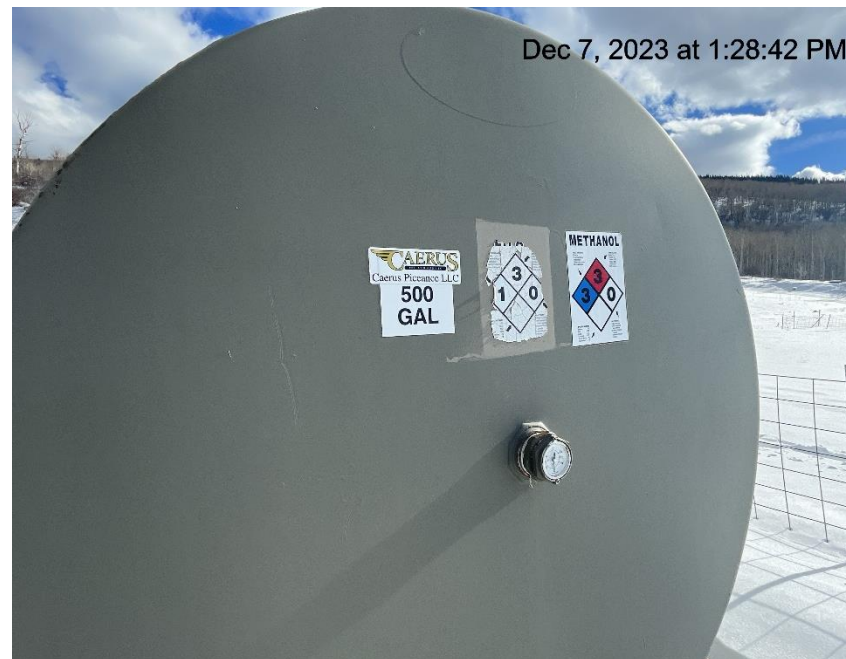
Photo # 8884 Methanol tank improperly labeled/lacks required information
