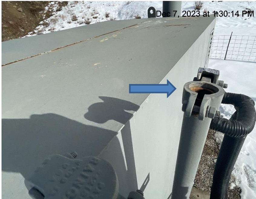
Photo # 8887 PRV vent line lacks cap
