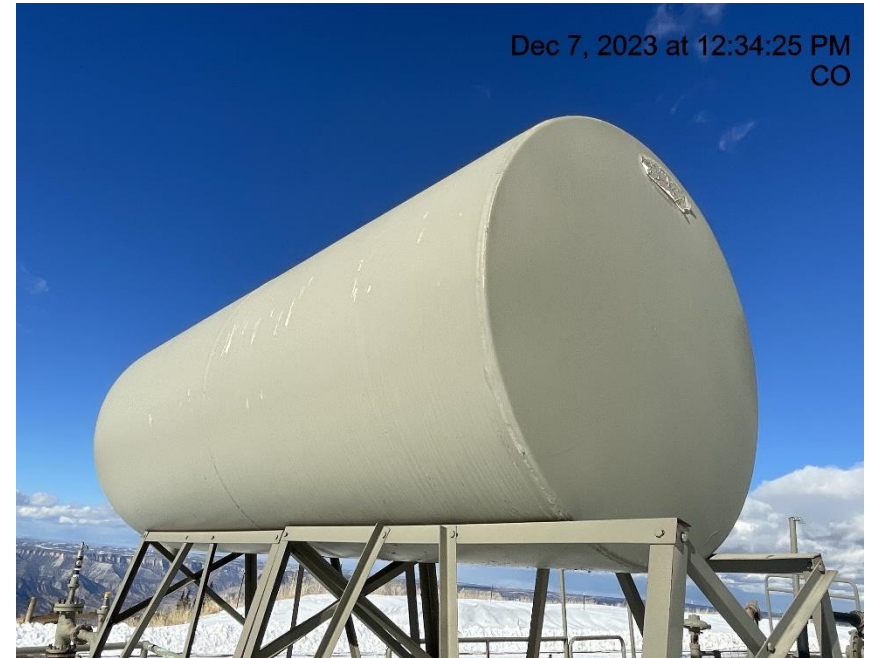
Photo # 8815 Methanol tank (next to production separators)
