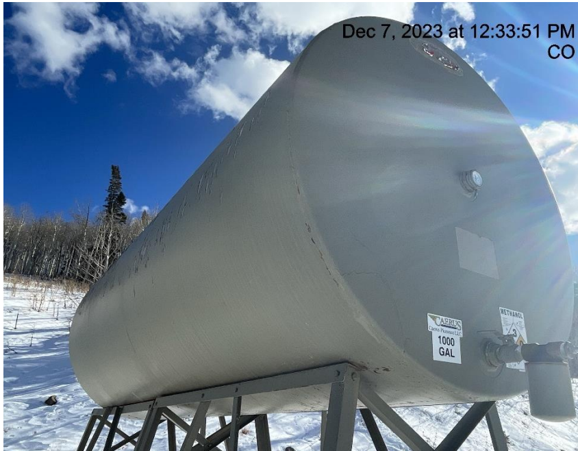
Photo # 8814 Methanol tank improperly labeled/lacks required information (next to production separators)
