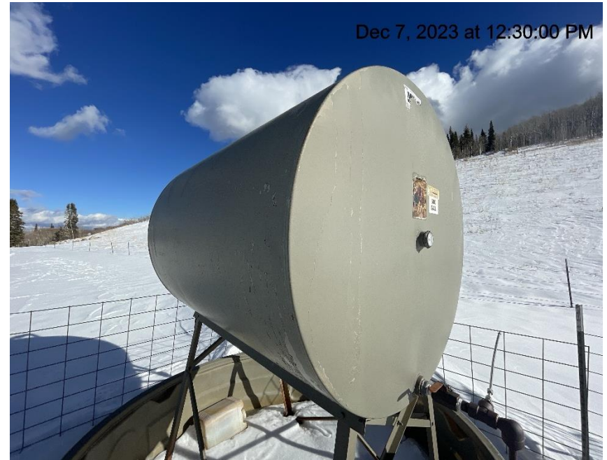
Photo # 8811 Methanol tank label weathered & illegible/ tank improperly labeled/lacks required information (near wellheads)
