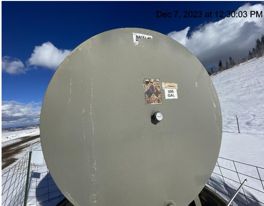
Photo # 8812 Methanol tank label weathered & illegible/ tank improperly labeled/lacks required information (near wellheads)
