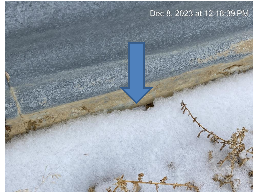
Gap below tank berm has not been resolved
