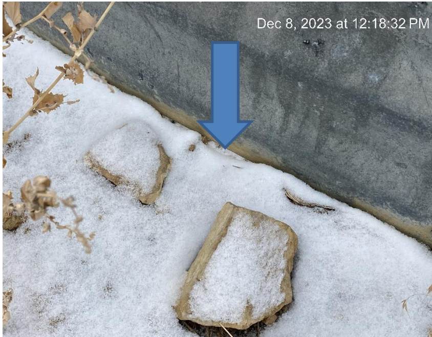
Gap below tank berm has not been resolved
