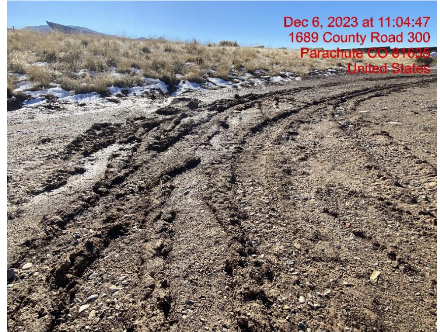
Lack of Stabilization – Photo #07995
