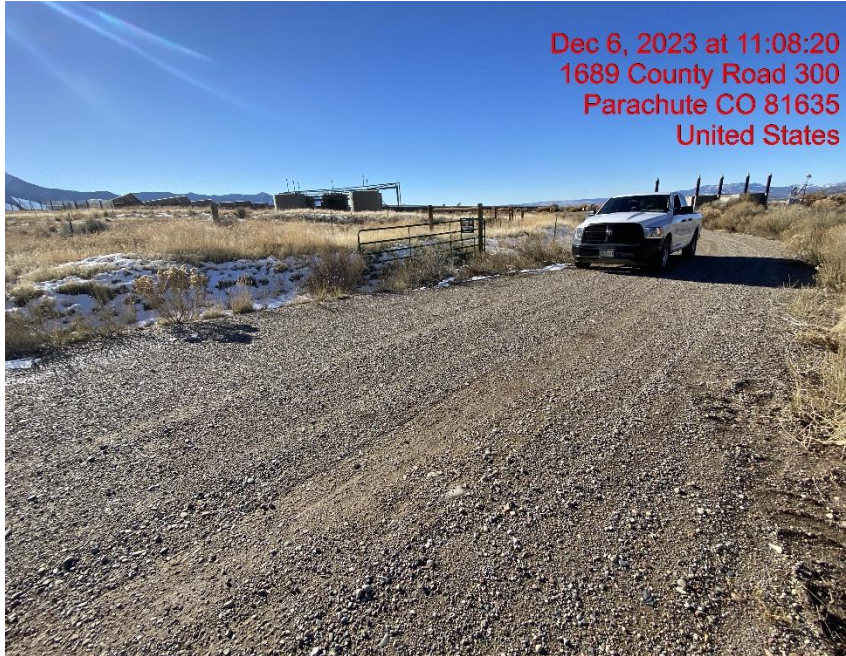
Insufficient Vehicle Tracking BMPs at Location Entrance/Exit – Photo #07998
