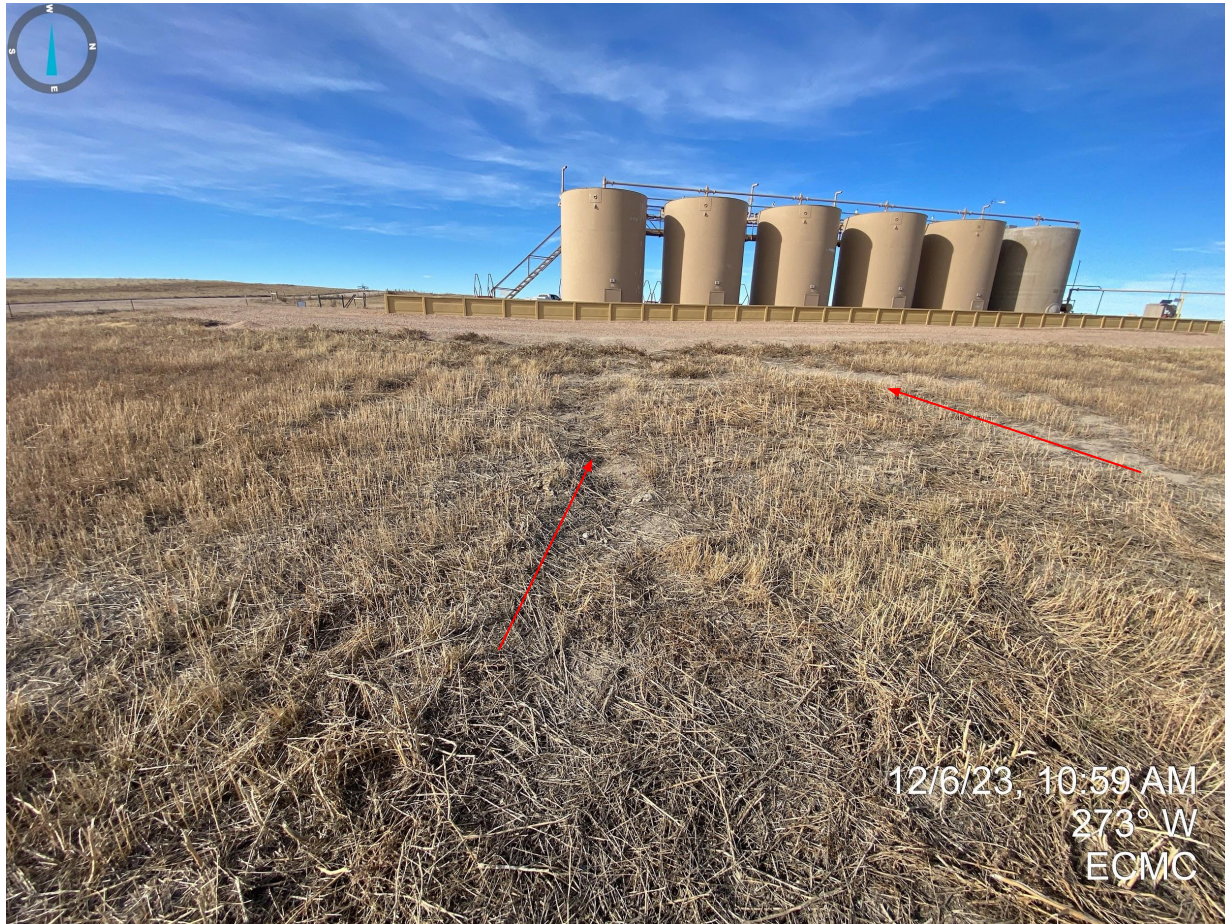
Photo 1. Taken from the east side of the location. Erosion degradation (e.g. rilling) is occurring from the production areas and is depositing sediment into the interim areas. Additional stormwater control measures are required in order to prevent further erosion degradation.
