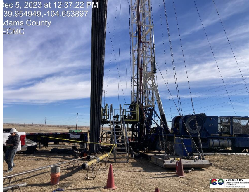
Pic 1 Rig / wellhead
