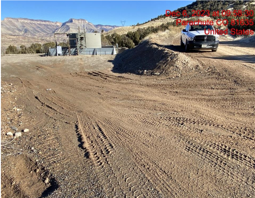
Insufficient Vehicle Tracking BMPs at Location Entrance/Exit – Photo #07946
