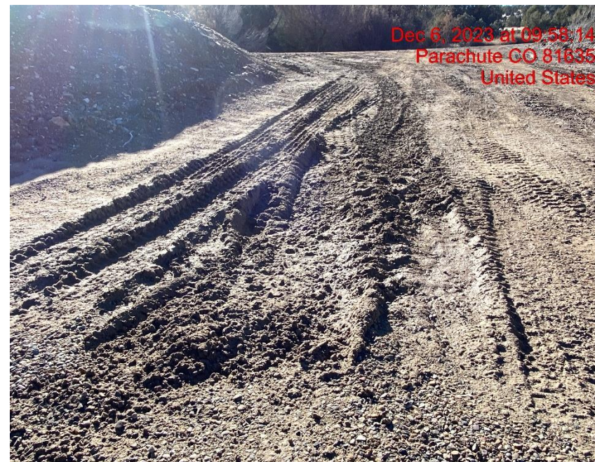
Lack of Stabilization – Photo #07945
