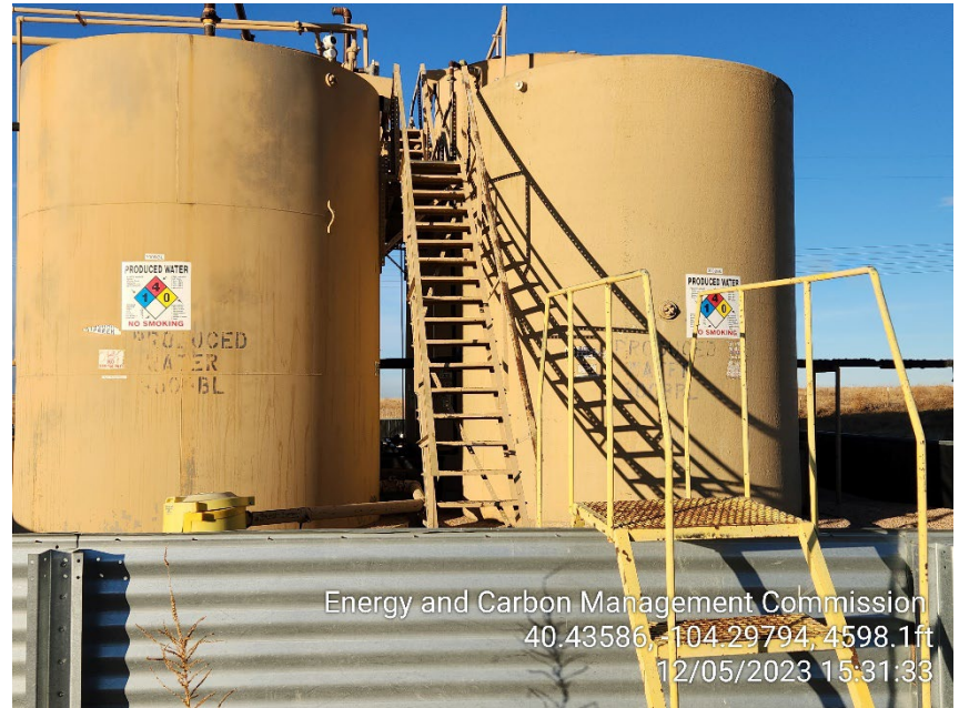
Photo 2 – Water Tank Labels have been installed
