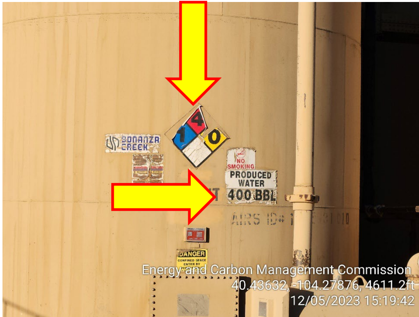
Photo 5 – Produces Water Tank Labels faded no longer visible
