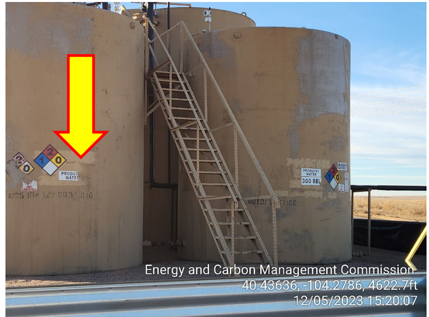
Photo 6 – Produces Water Tank Labels faded no longer visible
