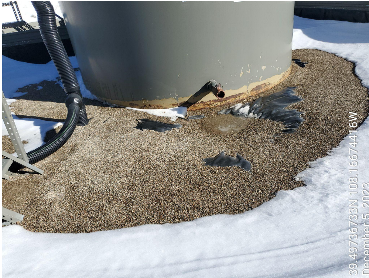
Photo 3: Tank loadline not capped/plugged.
