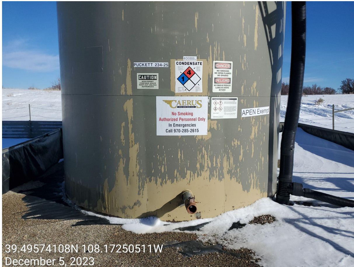
Photo 2: Tank loadline not capped/plugged.
