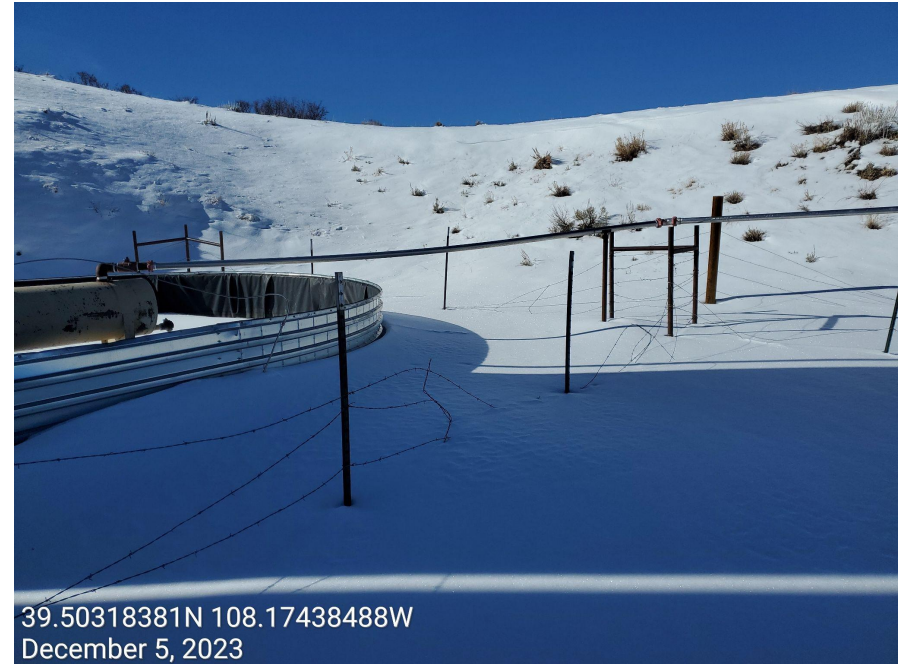
Photo 3: Fencing at separator equipment and tank battery facility in disrepair.
