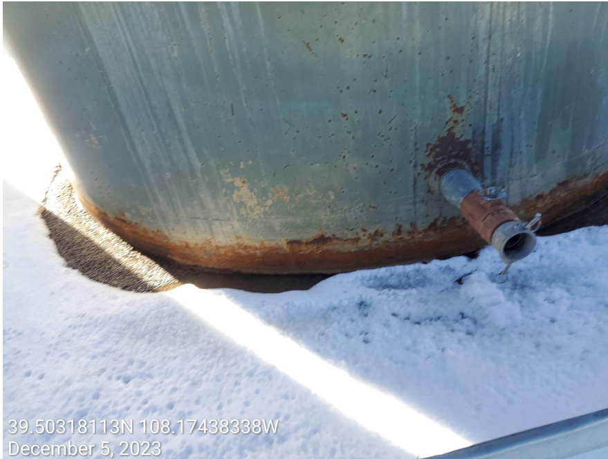
Photo 5: Tanks not capped/plugged.
