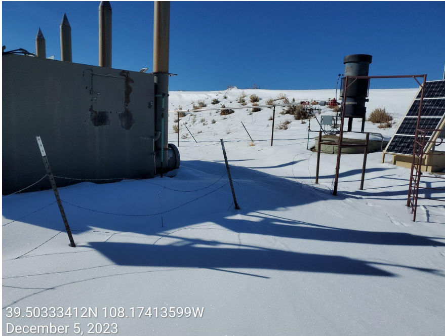
Photo 3: Fencing at separator equipment and tank battery facility in disrepair.
