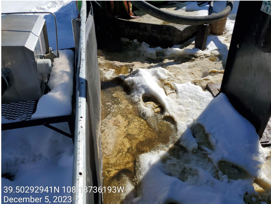
Photo 5: Produced fluids / spill observed within secondary containment at battery.
