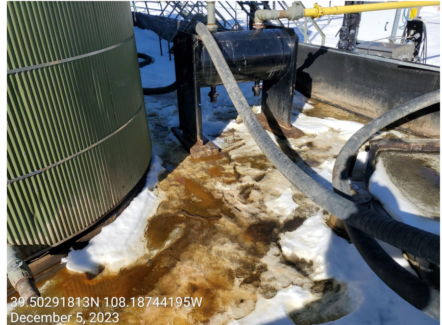
Photo 5: Produced fluids / spill observed within secondary containment at battery.
