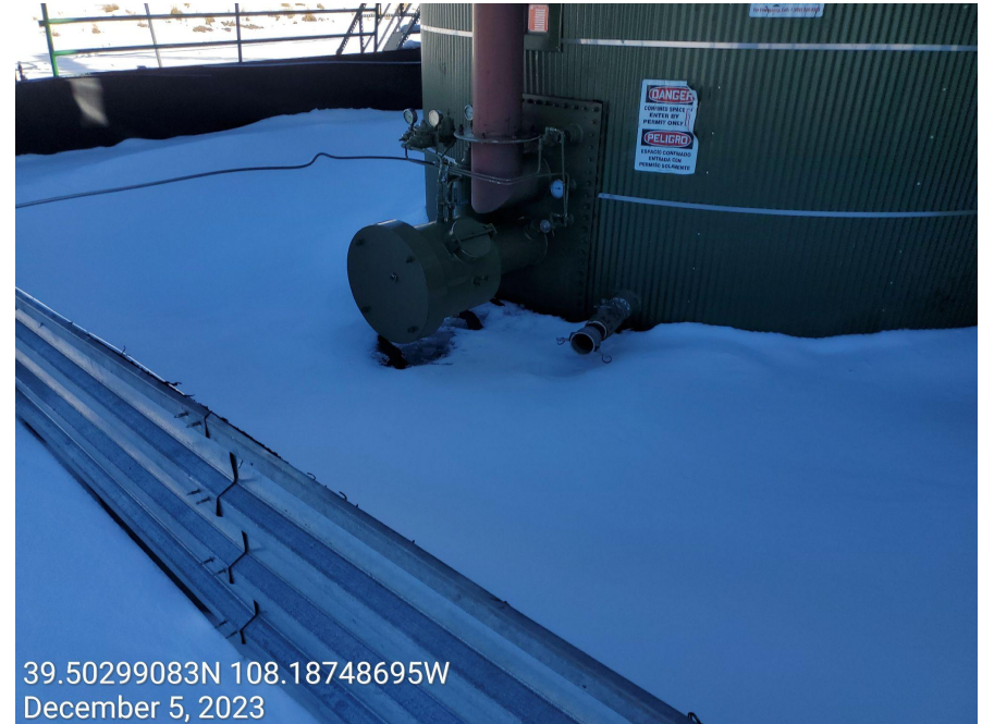
Photo 3: Photo example showing tanks at battery facility haven't been capped/plugged.
