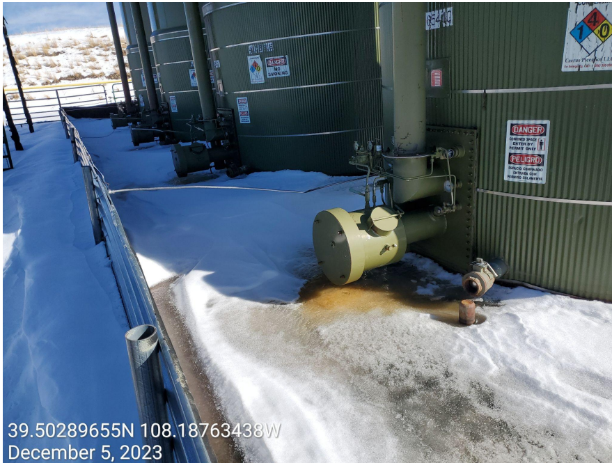
Photo 3: Photo example showing tanks at battery facility haven't been capped/plugged.
