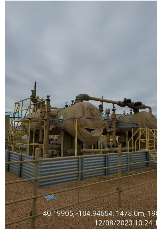
Photo 3 Horizontal Separators
