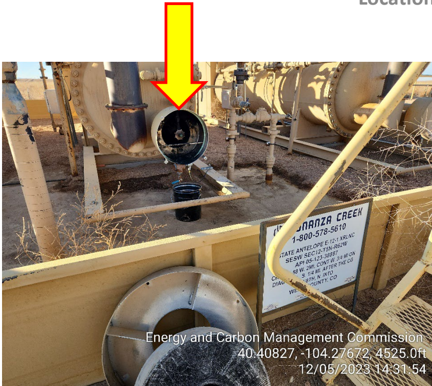
Photo 5 – Middle Separator open to Atmosphere
