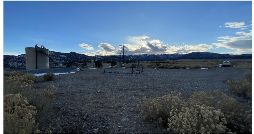
North East corner of location.
