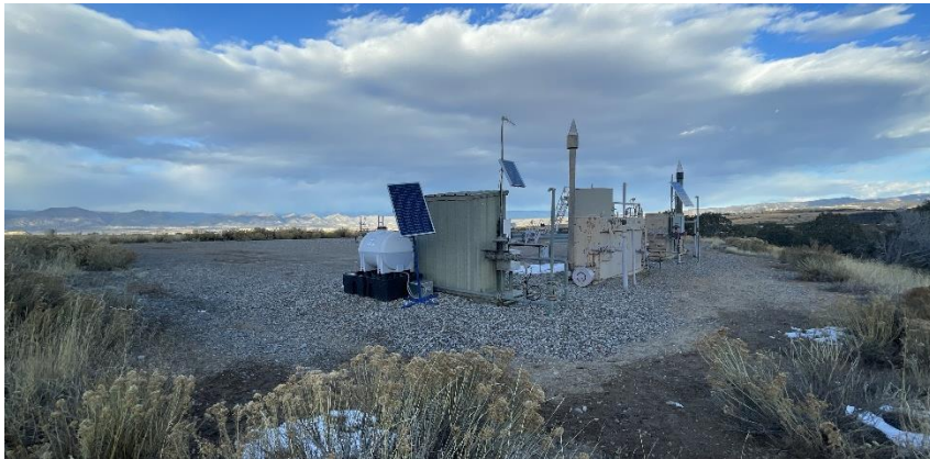
South West corner of location.
