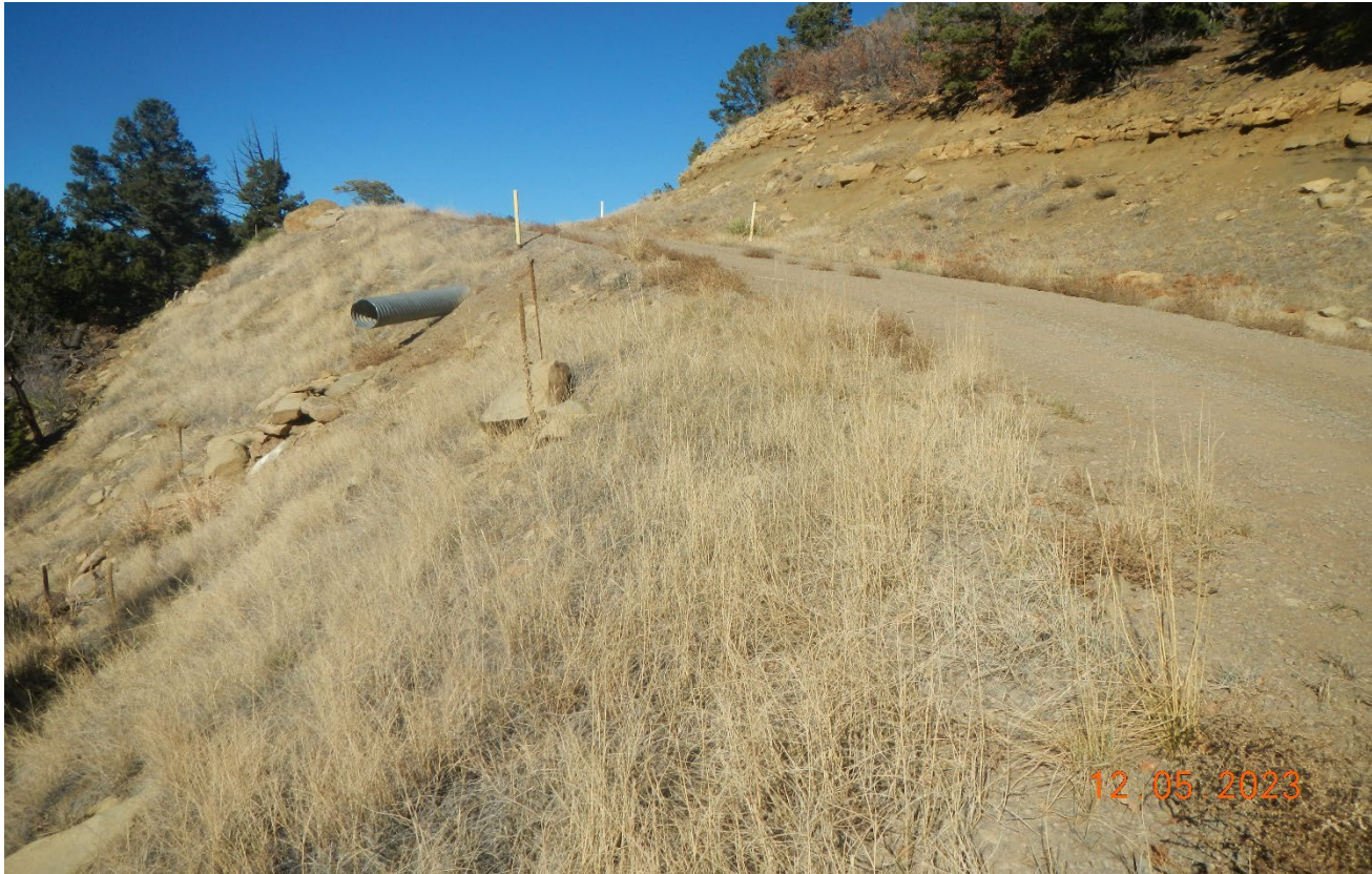
Photo 1. Facing northwest along the access road which is stabilized with vegetation and gravel. Culvert outlet protection is installed at the culvert outlet.
