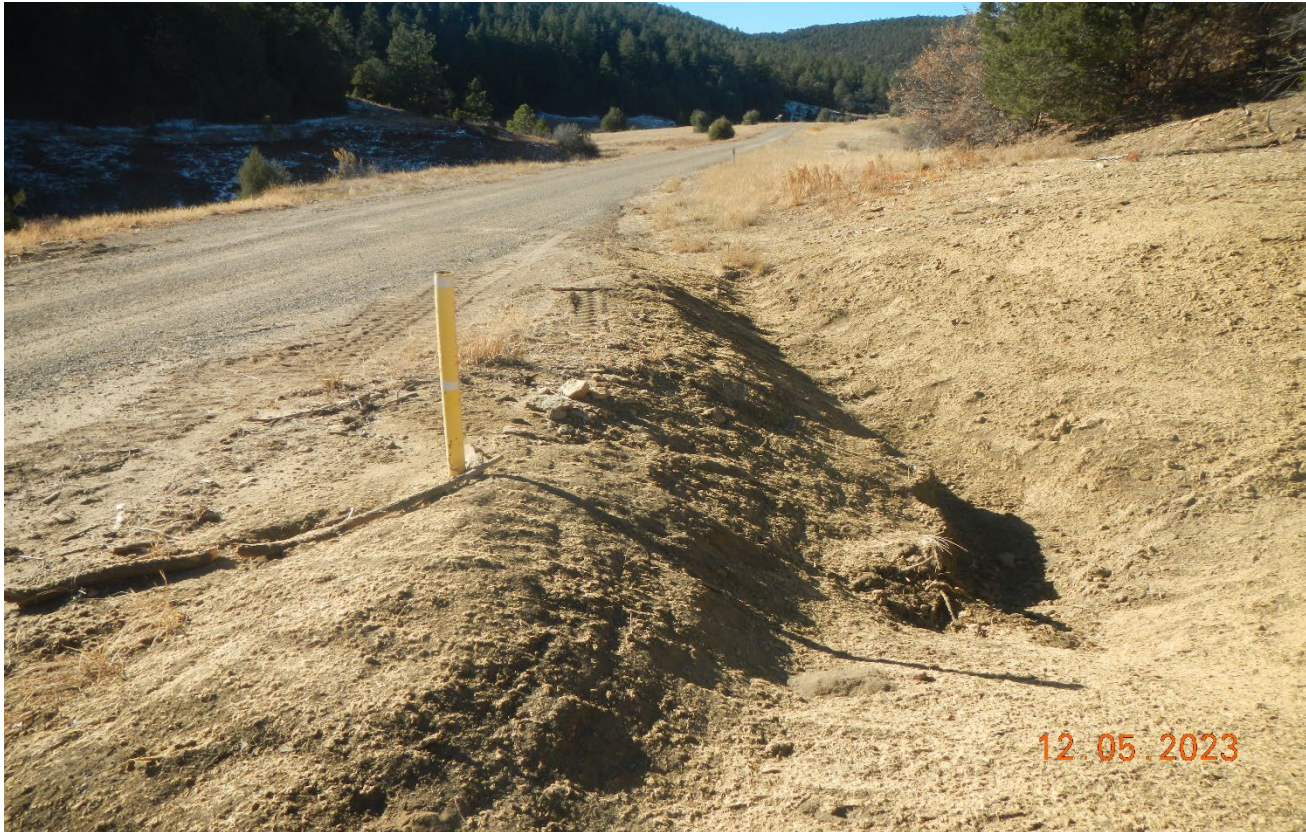
Photo 2. Facing west along the road. This culvert was repaired but additional cleanout will be needed. Lat/Long:37.14485,-104.03594.
