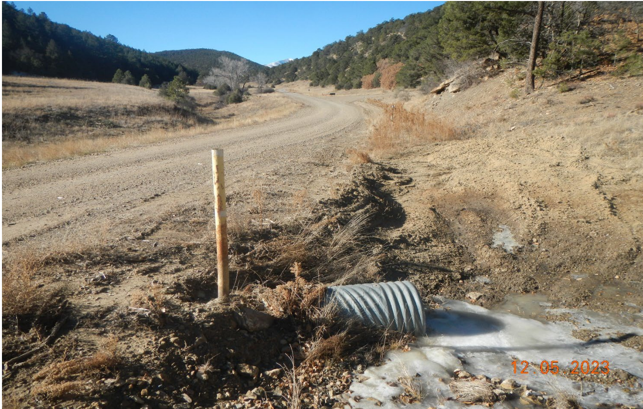
Photo 1. Facing west at the main access road. This culvert has been cleaned out and maintained.
