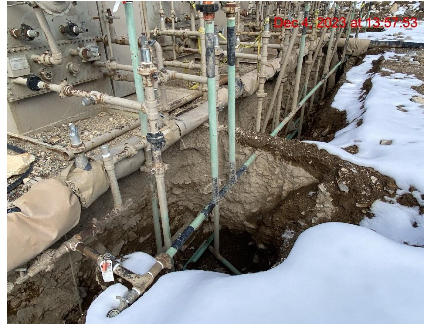
Open Trench at Separators – Photo #07915
