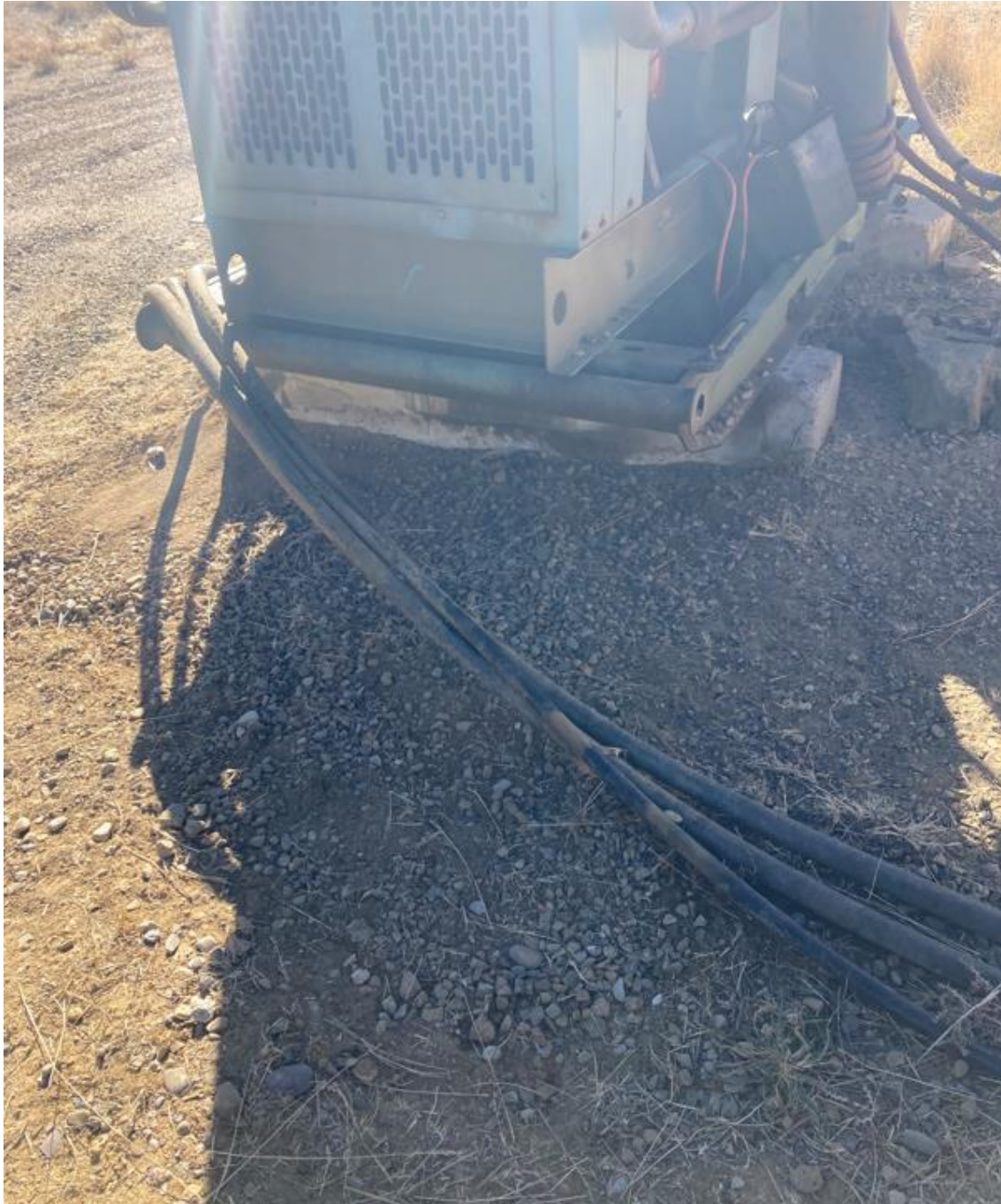
PHOTO 1: THE OILY FLUIDS HAVE BEEN REMOVED FROM THE ENGINE SKID AND MAINTENANCE HAS BEEN CONDUCTED ON ALL EQUIPMENT. THE IMPACTED SOIL HAS BEEN REMOVED AND REPLACED WITH FRESH GRAVEL MATERIAL. THE SELF INSPECTION PROCESS HAS BEEN REVIEWED.
