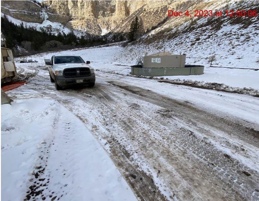
Insufficient Vehicle Tracking BMPs at Location Entrance/Exit – Photo #07835
