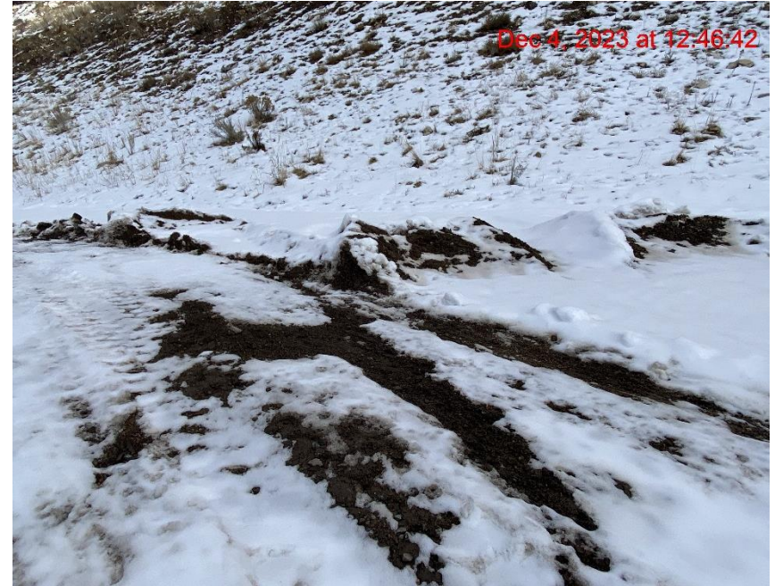
Lack of Stabilization/Sediment Transport of Sediment – Photo #07833
