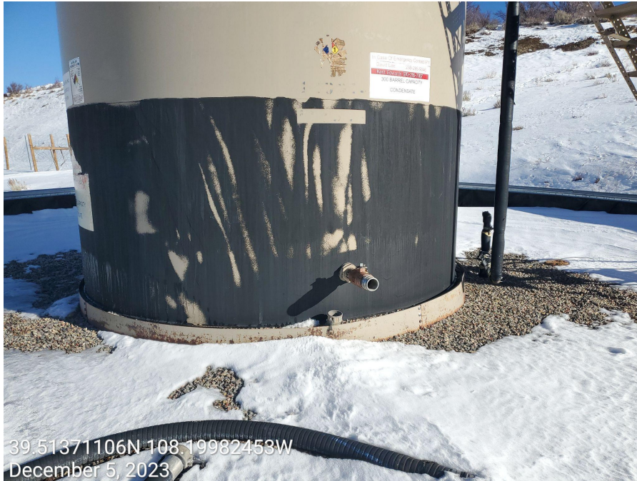
Photo 5: Caps/plugs missing from tanks.
