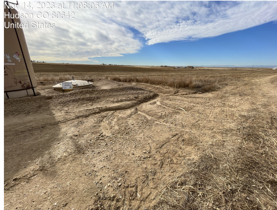
Photo 6. Photo of stormwater erosion on access road and around tank battery . Photo taken facing southwest.
