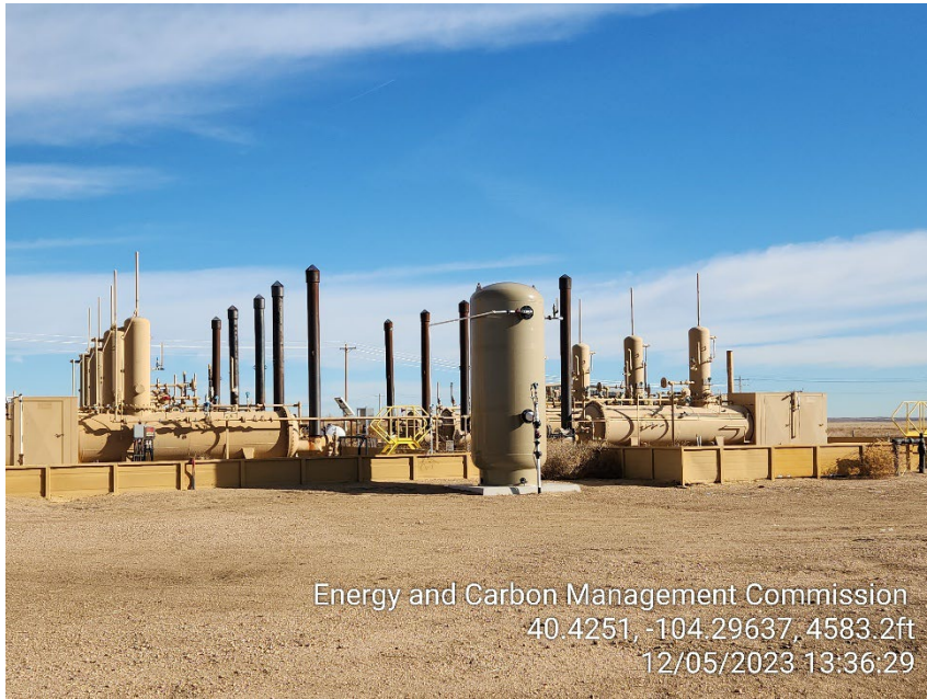
Photo 15 – Separators and Instrumental Air Unit
