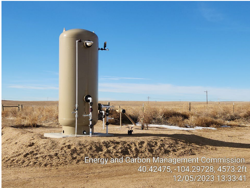
Photo 3 – Instrumental Air Unit
