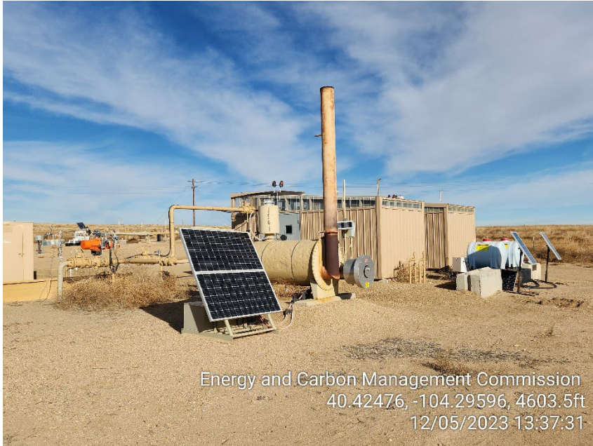
Photo 17 – Line Heater and Gas Lift Injection Meter Houses
