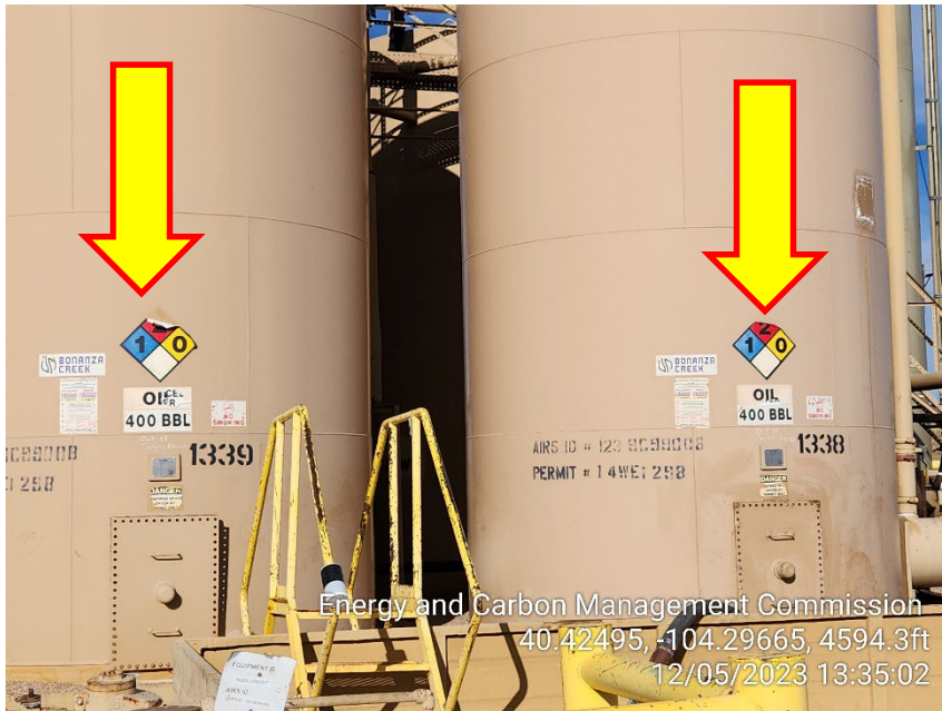
Photo 11 – NFPA Labels on 1339 and 1338 Tanks
