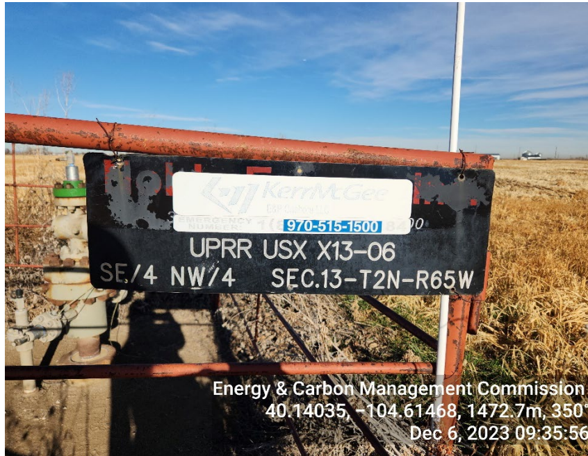
Photo 5: Wellhead Sign, Operator Name no longer visible
