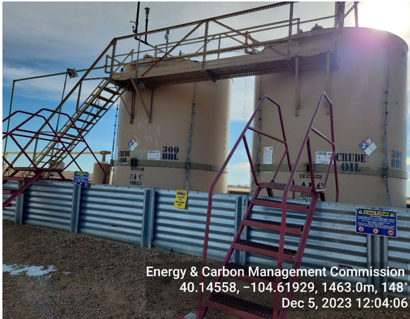
Photo 3: Centralized tank battery
