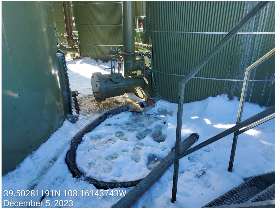
Photo 4: Photos examples showing tanks lack caps/plugs
