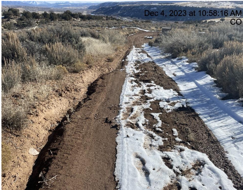
Photo # 8265 Degradation, erosion & transport of sediment on lease road
