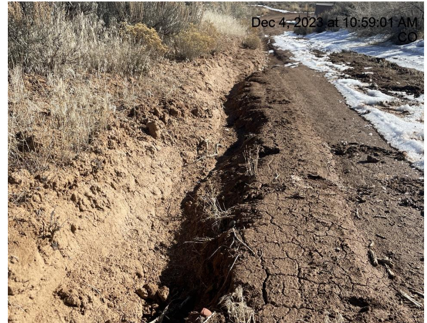
Photo # 8268 Degradation, erosion & transport of sediment on lease road
