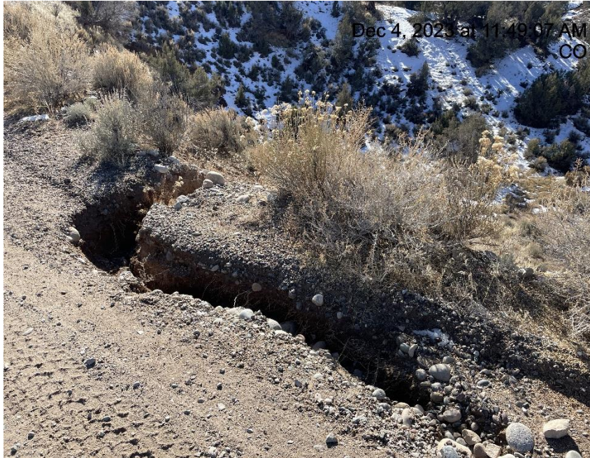
Photo # 8269 Erosion & transport of sediment on lease road
