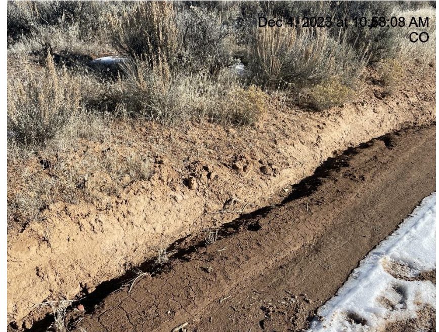
Photo # 8264 Degradation, erosion & transport of sediment on lease road
