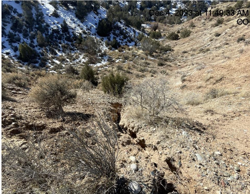
Photo # 8275 Erosion & transport of sediment off lease road & going down slope
