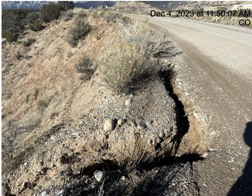
Photo # 8271 Erosion & transport of sediment on lease road & going off lease road & down slope
