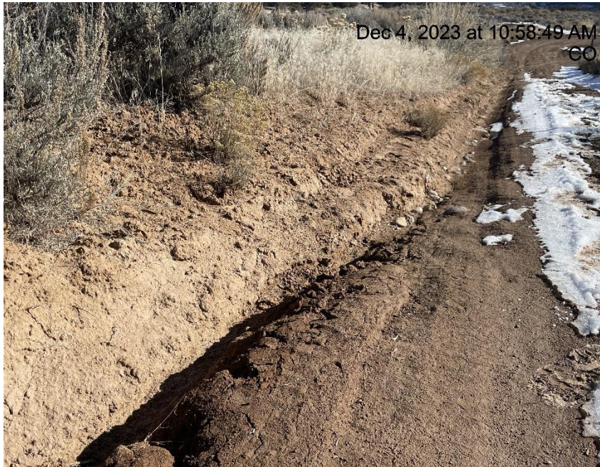
Photo # 8267 Degradation, erosion & transport of sediment on lease road
