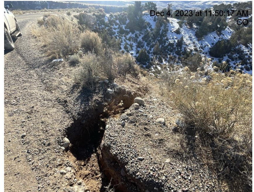
Photo # 8272 Erosion & transport of sediment on lease road & going off lease road & starting to go down slope
