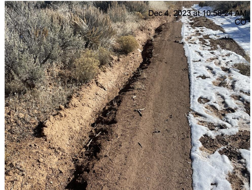
Photo # 8266 Degradation, erosion & transport of sediment on lease road
