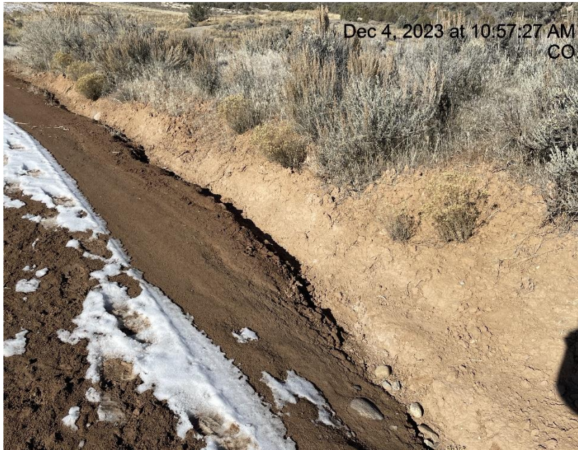
Photo # 8261 Degradation, erosion & transport of sediment on lease road
