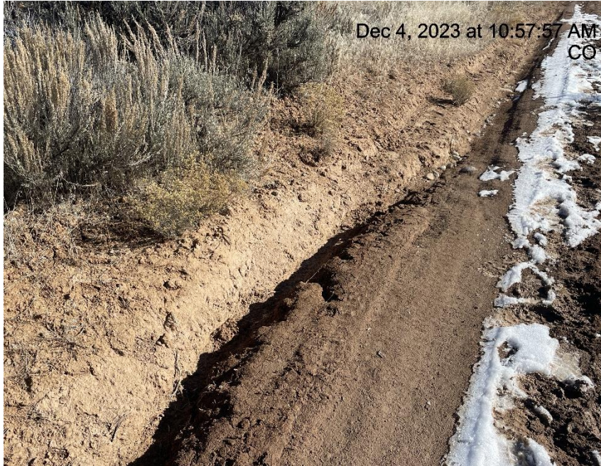
Photo # 8263 Degradation, erosion & transport of sediment on lease road
