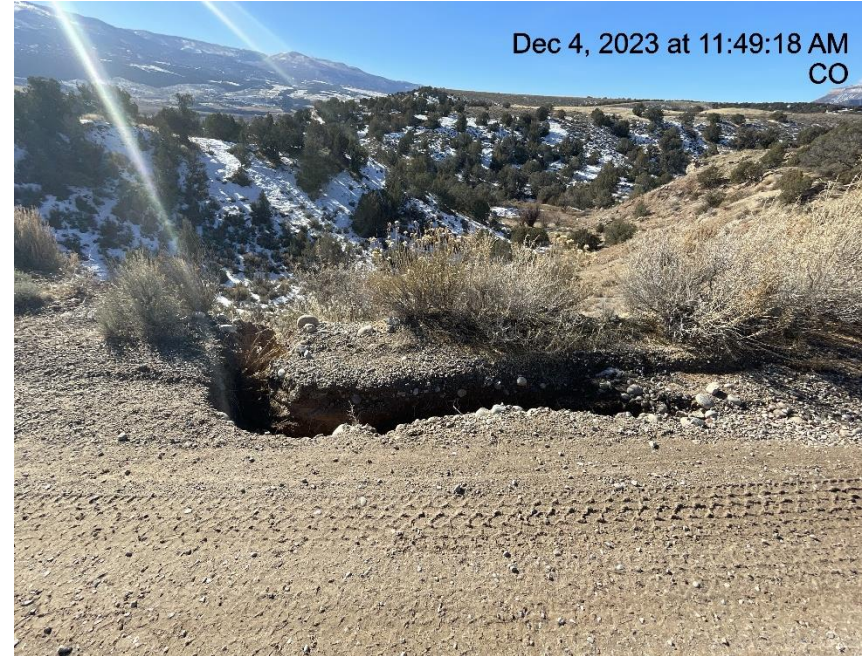
Photo # 8270 Erosion & transport of sediment on lease road
