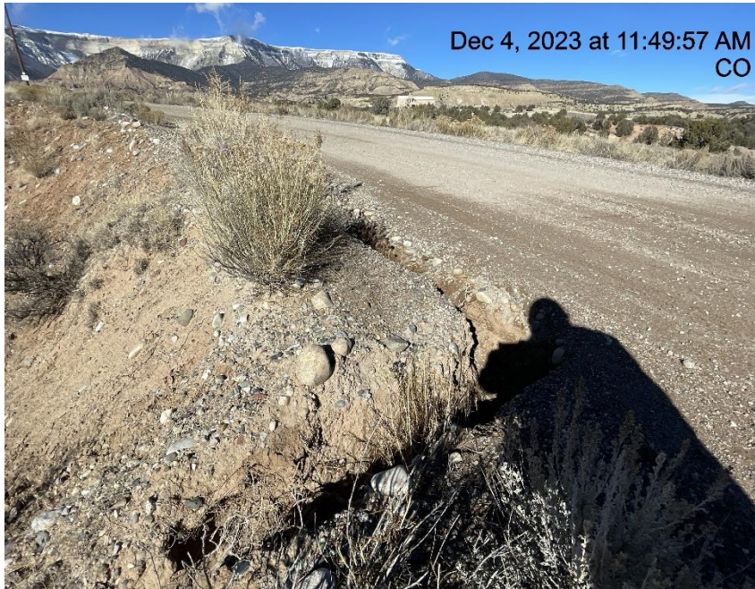
Photo # 8273 Erosion & transport of sediment on lease road & going off lease road & down slope
