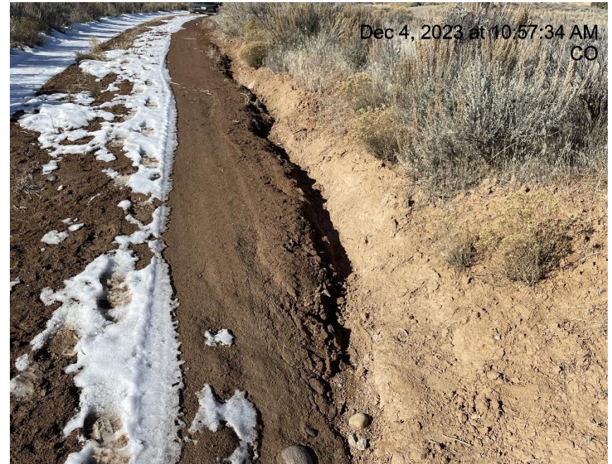
Photo # 8262 Degradation, erosion & transport of sediment on lease road
