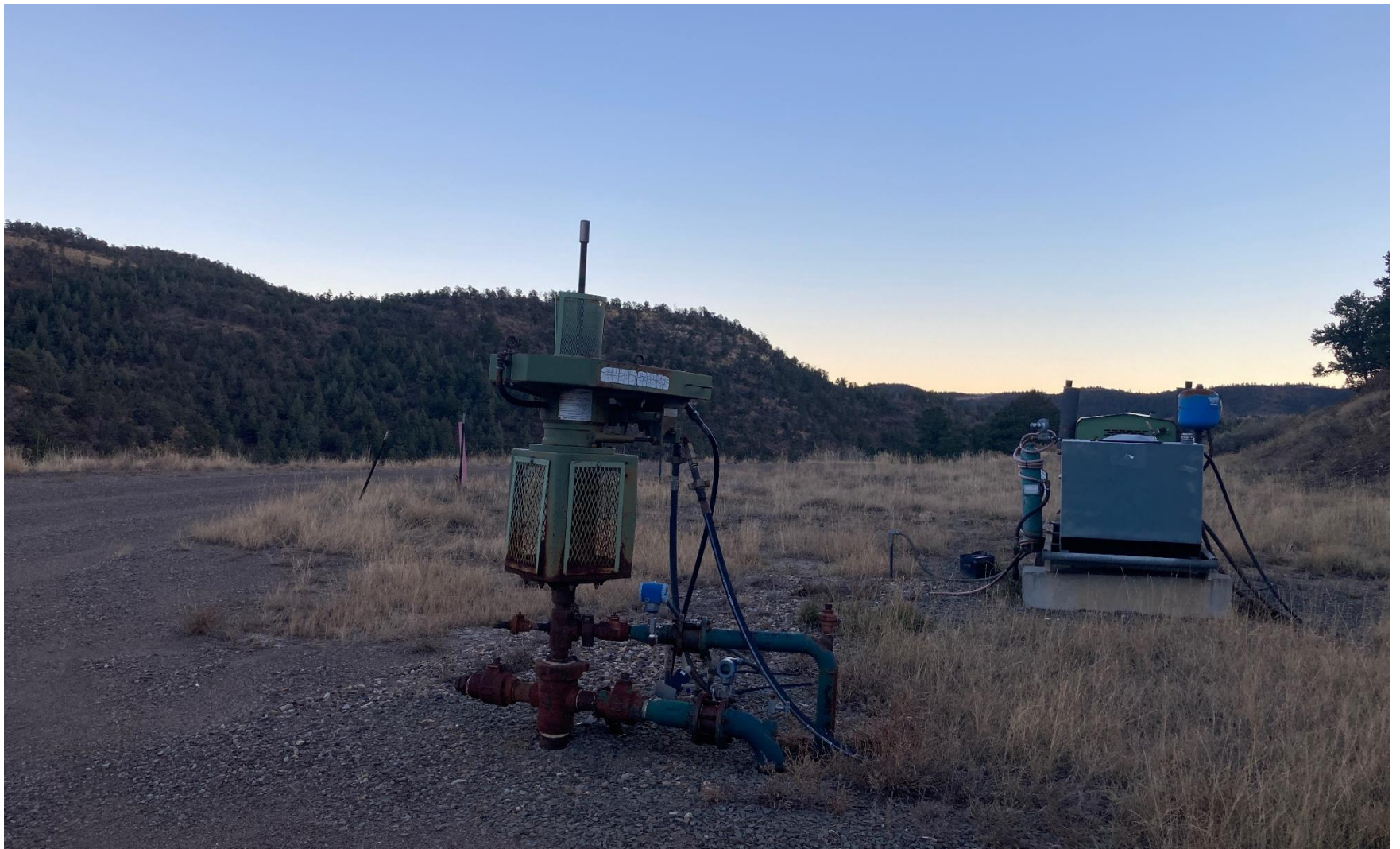
PHOTO 3: WELLHEAD AND EQUIPMENT
