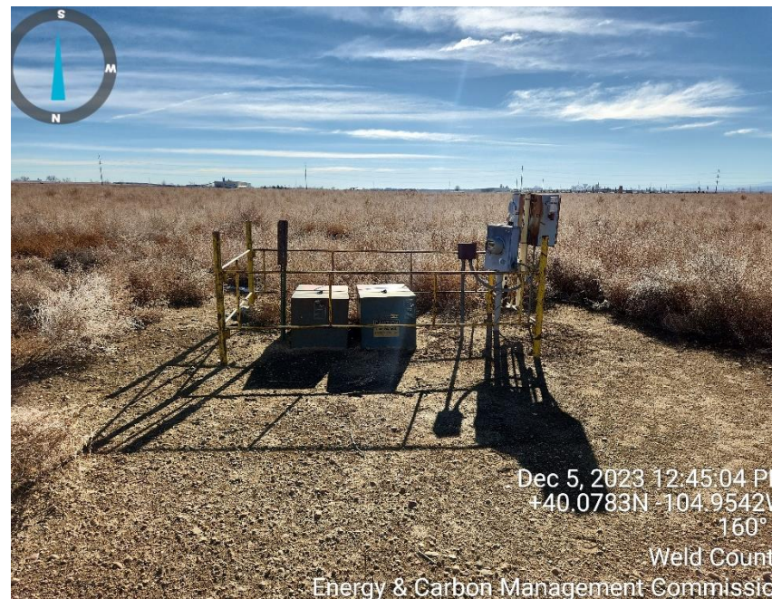
Photo 2 electrical disconnect panel
