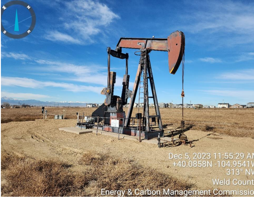
Photo 1 well head and equipment
