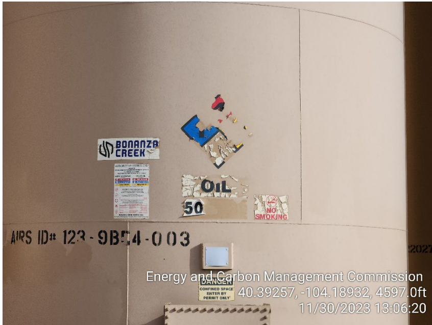
Photo 11 – Center Tank – NFPA, Content and Capacity Labels
