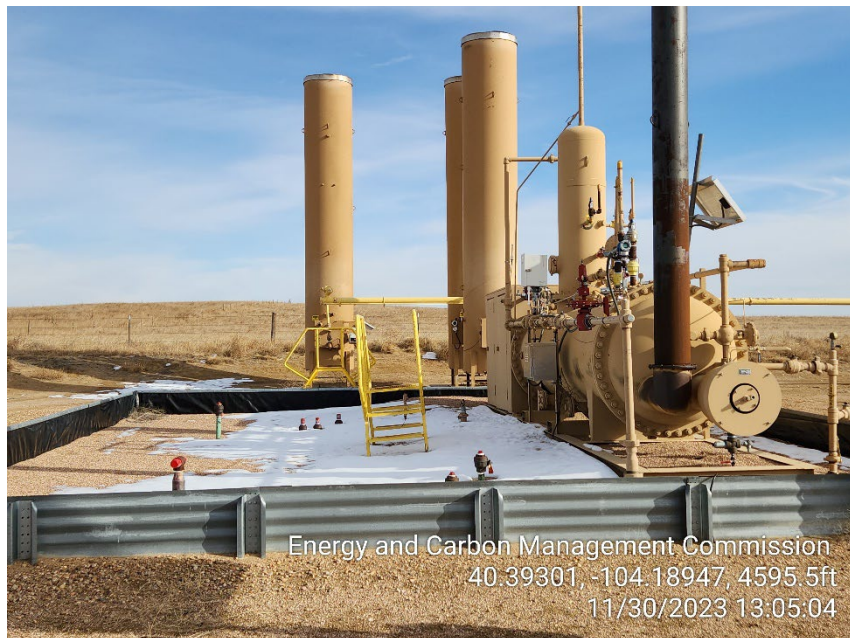
Photo 5 – Separators and ECDs
