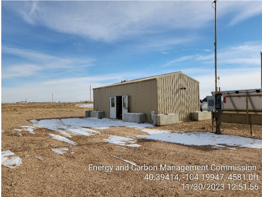
Photo 3 – Gas Lift Meter Injection House
