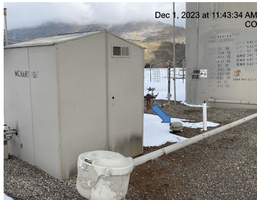
Photo # 8207 Thief hatch/unknown buried tank in tank battery containment/tank not labeled
