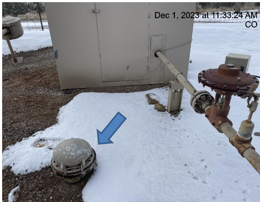
Photo # 8206 Thief hatch/unknown buried tank in tank battery containment/tank not labeled
