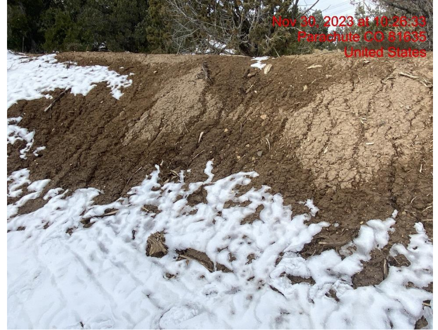
Insufficient Erosion Control – Photo #07792
