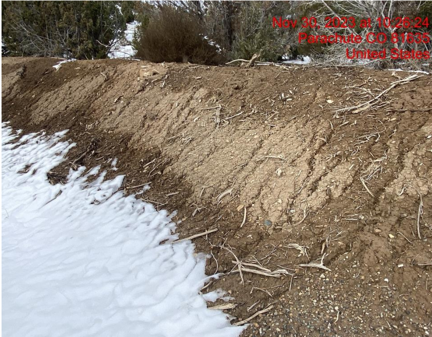
Insufficient Erosion Control – Photo #07791
