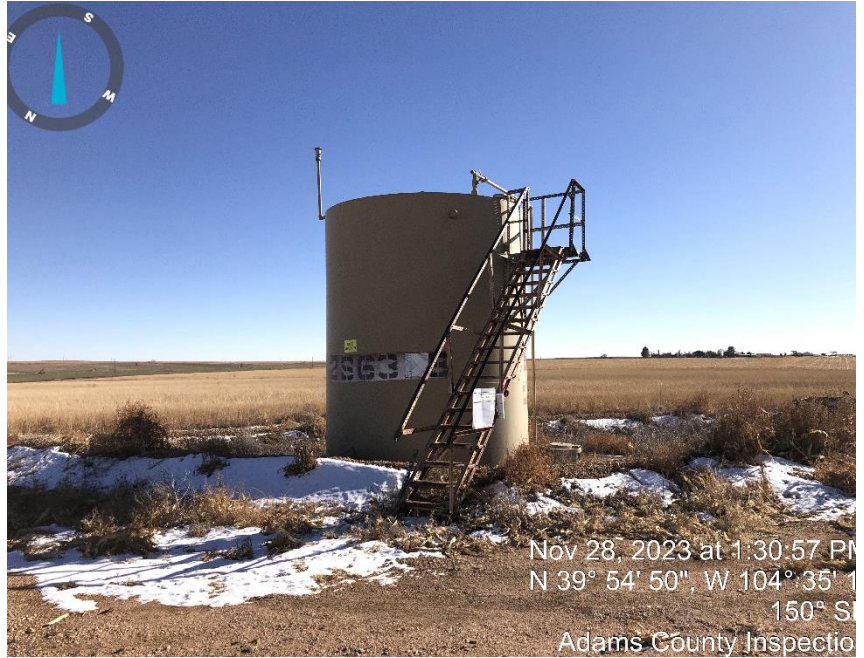
Photo #2 Crude tank.
