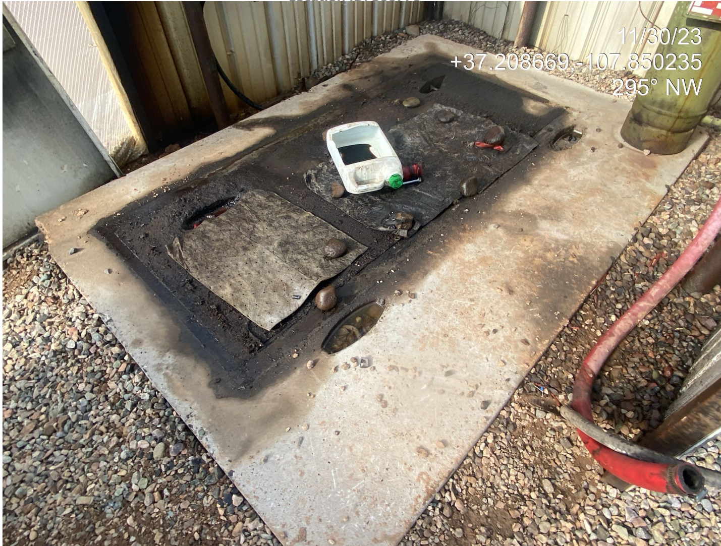
Photo 2. View of oily substance in plastic container and spilling over onto concrete pad.
