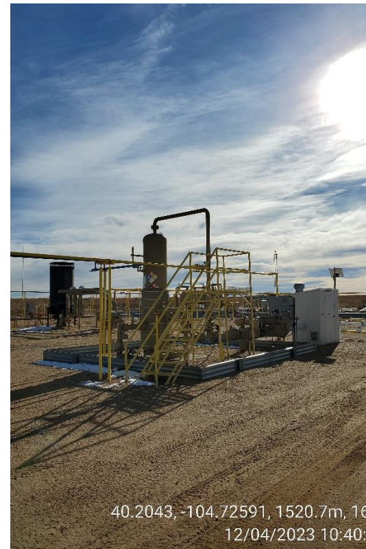
Photo 3 Vertical Separator
