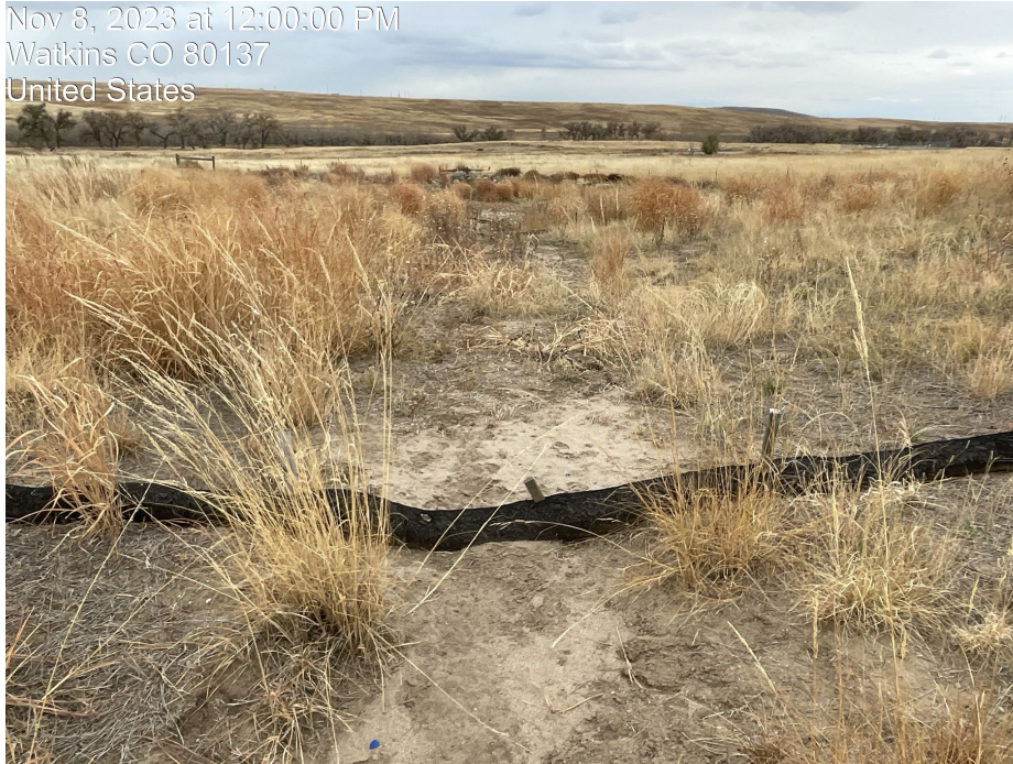
Photo 5. Photo taken of interim reclaimed area of improperly installed wattle. Photo taken facing northwest.
