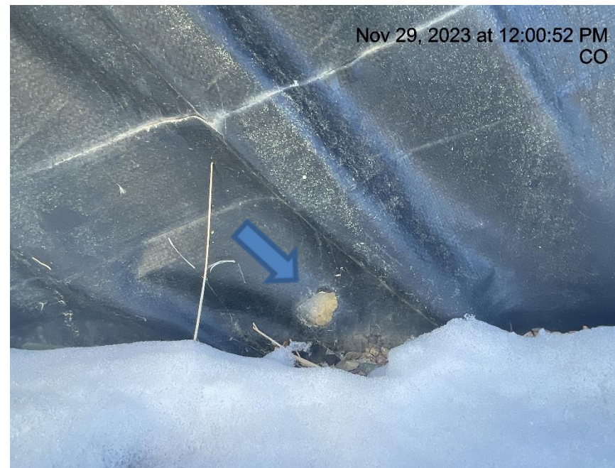
Photo # 7844 Hole in liner/liner needs maintenance
