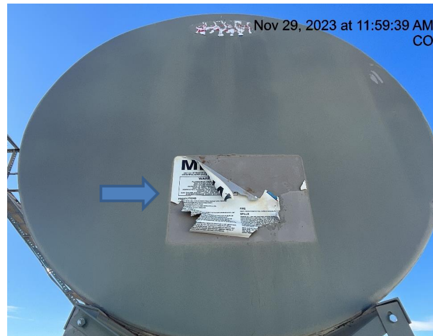
Photo # 7840 Tank label damaged & illegible
