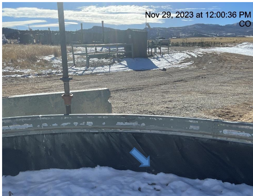
Photo # 7843 Hole in liner/liner needs maintenance
