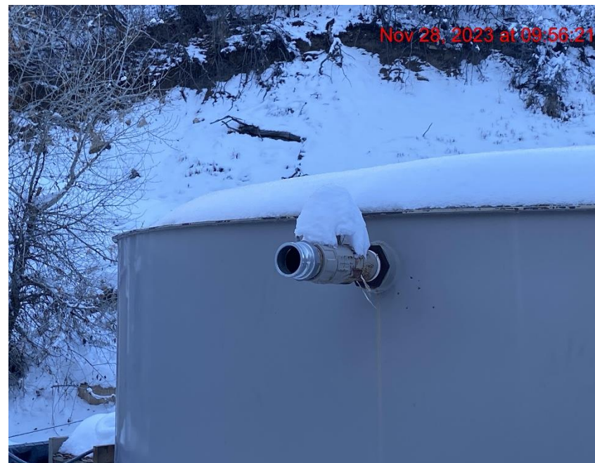
Open-Ended Vent/Load Line – Photo #07717
