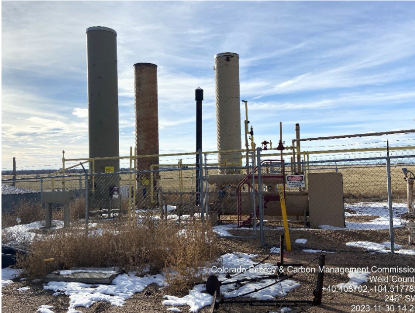
Photo #3 Trebor B 11-25 Battery site Inactive | Shut-down ECD(s), Separator(s)
